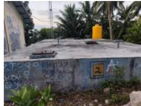
Reservoir Wutik 1, Koting
